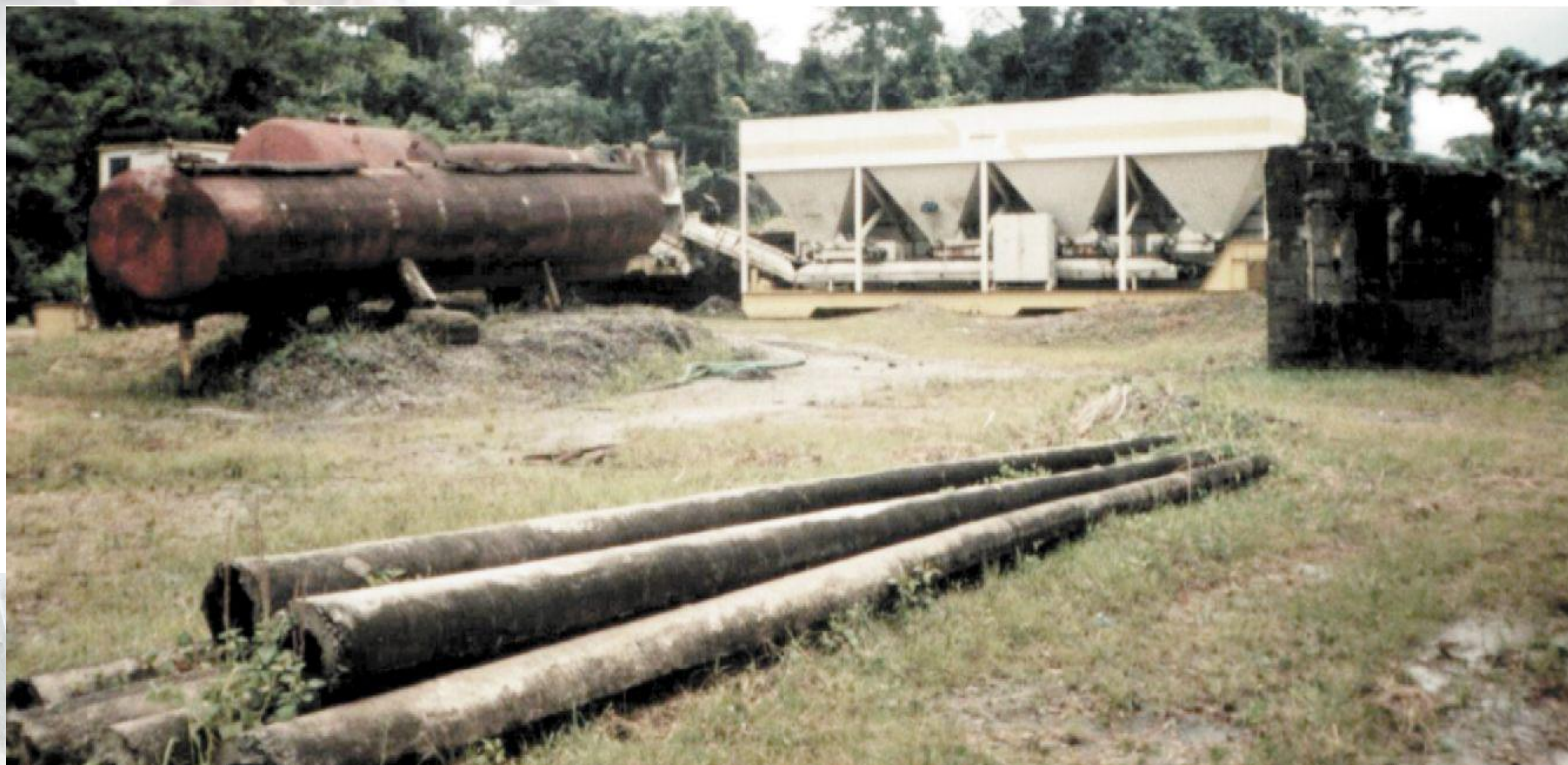
Abandoned Rural Electrification Project : Kanyang, Cross River
